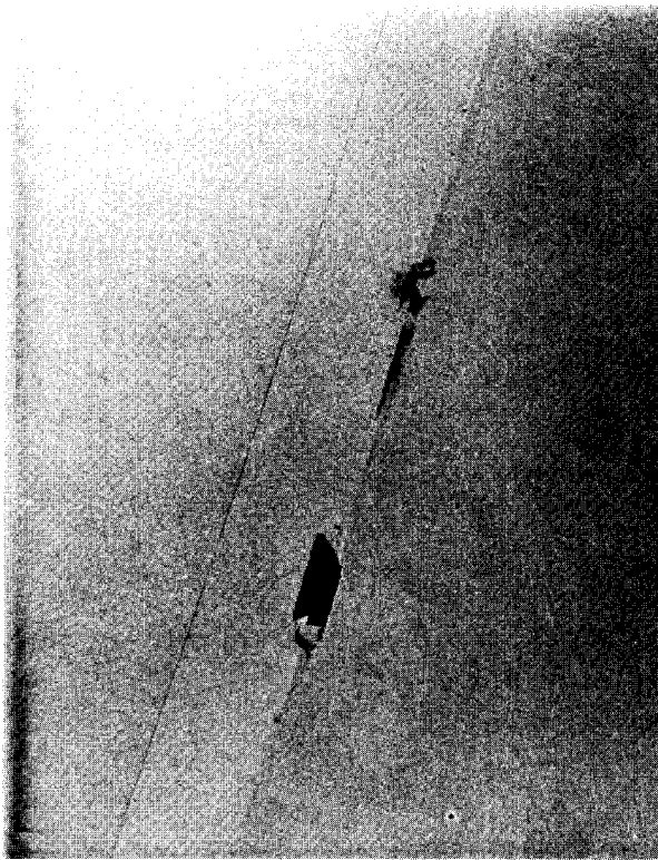
FIG. 6--Detail of Scotchlite tear.
