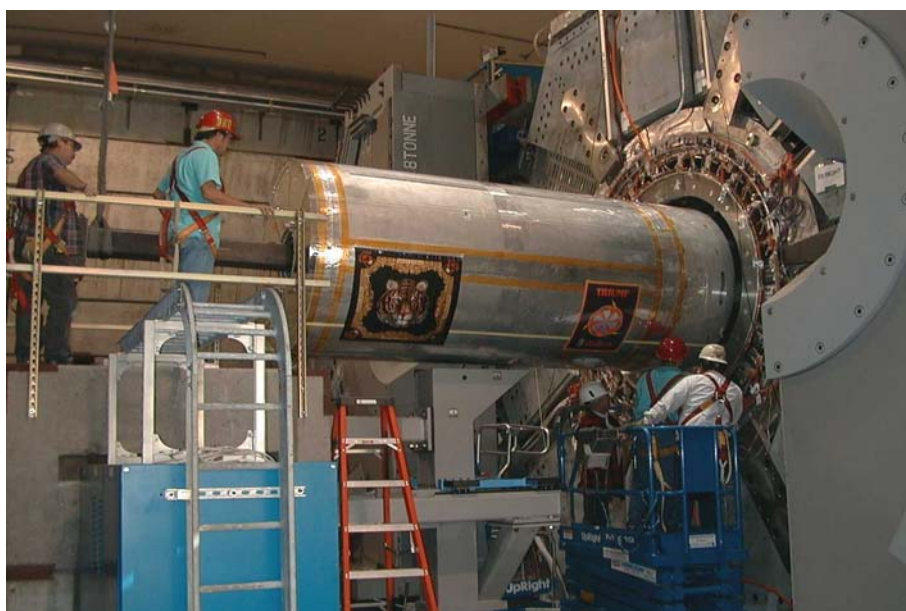
Figure 2.14: DCH installation (August 1998).
