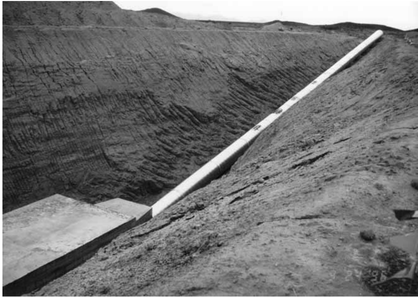
Fig. 15. The Palo Verde underground laboratory at the time of construction (Fall 1996).
