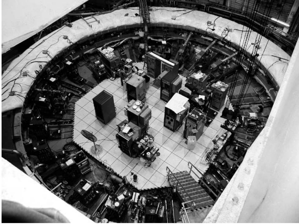
Fig. 5. The 700 ton muon (g - 2) storage ring during a maintenance period. The magnet yoke is covered with (white) thermal insulation, except at 9:00 o'clock where it is pulled back. The lighter colored inner-radius ring at 9:00 is the top cryostat for the inner-radius coil, and the bottom inner-radius cryostat can also be seen below the magnet gap at 2 o'clock. Most of the 24 electron calorimeter stations are installed. The muon kicker modulators are the three "cannon-like" objects at 1:00 o'clock. Two sets of tracks the detectors ride on can be seen to the right of the third kicker modulator, since these detectors have been removed.
