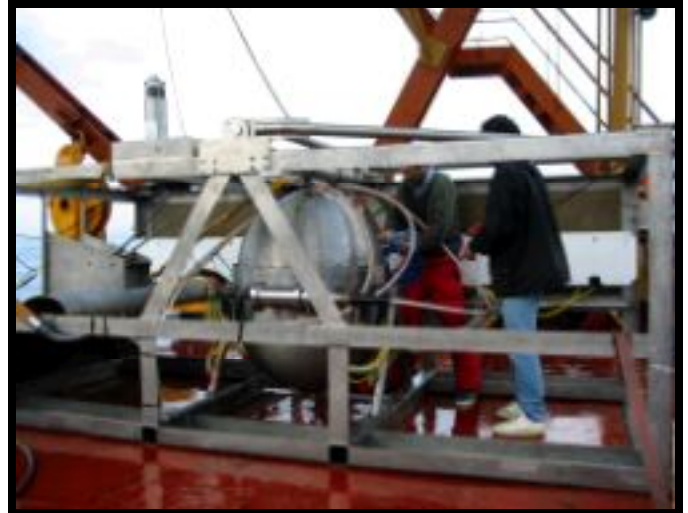
Fig. 20b Antares junction box during deployment; illustrating acoustic transponder (top) titanium support frame and undersea cable attachment.
