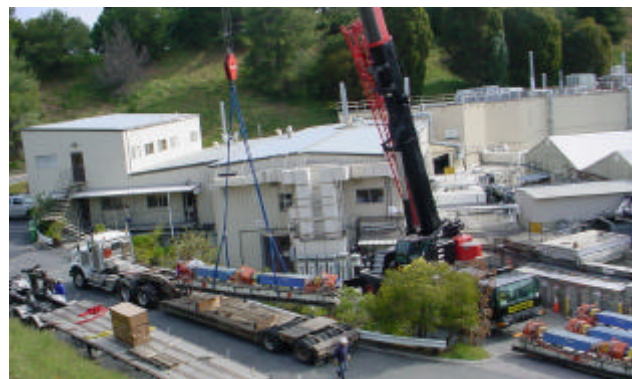
Figure 1: Removal of SPEAR 2 magnet/chamber girders.
