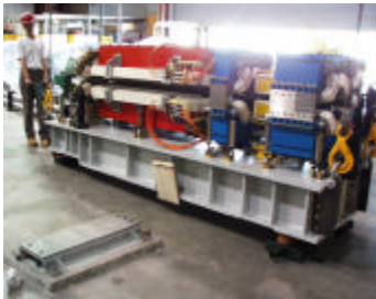
Figure 2: Magnet raft on installation rollers. Grouted mounting plate in foreground.
