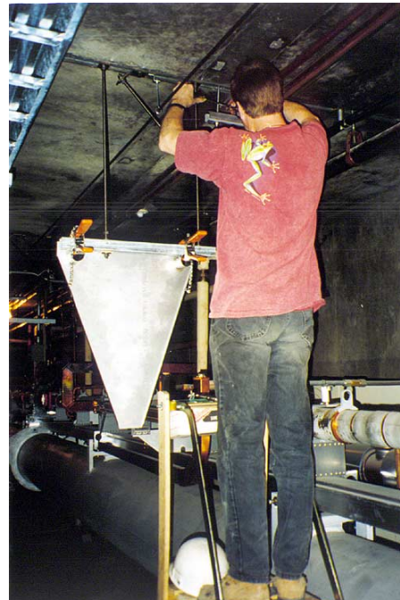
Fig. 6 Bypass chamber support installation
