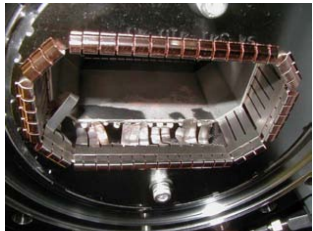
Figure 6: Damaged rf shield of a bellows unit.
