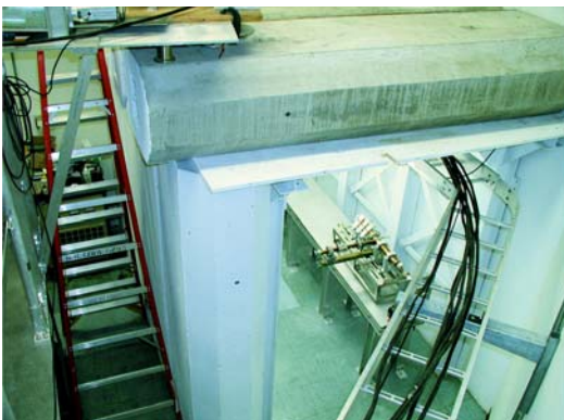
Figure 3: Photograph of concrete bunker, showing accelerator table and 5-MeV injector.
