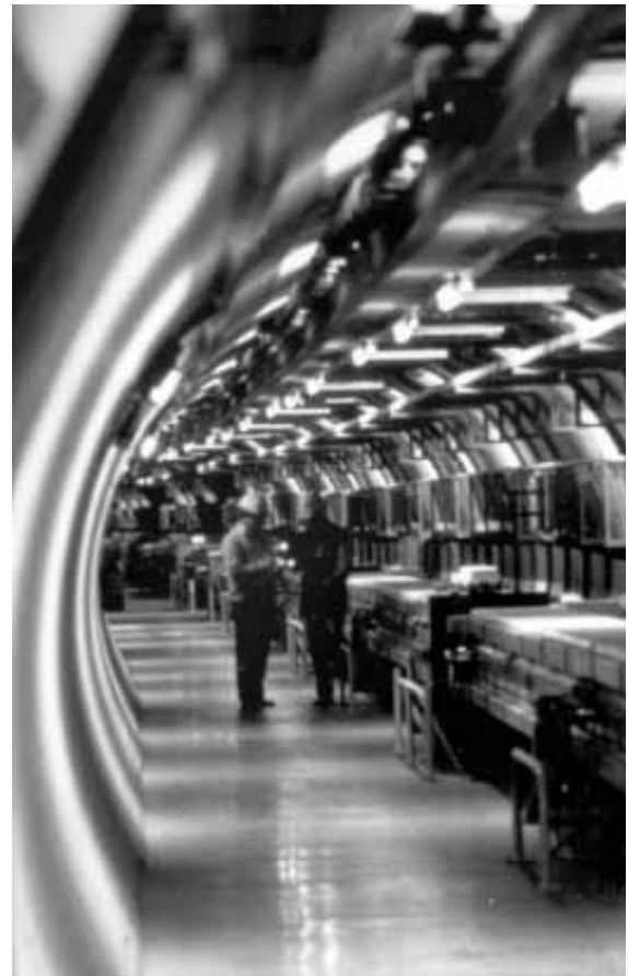
The LEP tunnel at CERN which houses the most powerful electron/positron collider and will eventually house the Large Hadron Collider, which will be able to recreate conditions that last existed 10^{-15} seconds after the Big Bang. (Courtesy CERN)
