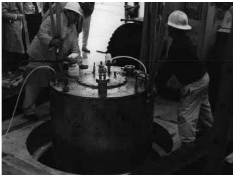
The magnet cryostat being installed at Lawrence Livermore National Laboratory in spring 1995.
