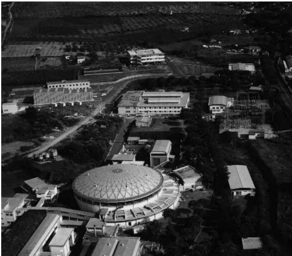
The site and the buildings that will house DAΦNE and its detectors. The ferro-concrete single span dome, designed by Pier Luigi Nervi, a famous Italian architect, is a national landmark.
