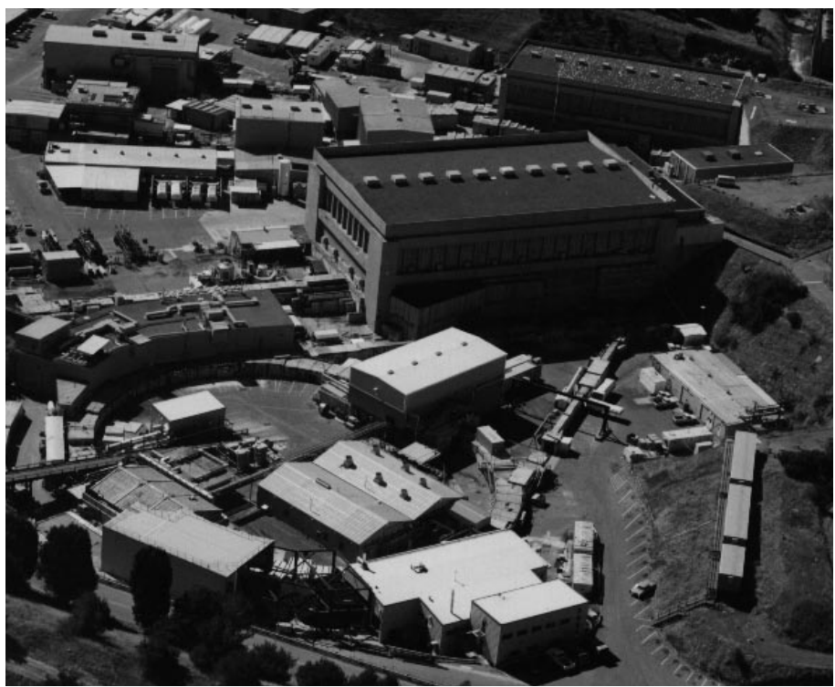
Aerial view of the Stanford Synchrotron Radiation Laboratory at SLAC.
