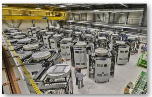
Figure 3 CERN SPS Thales Solid State Power Amplifiers,
