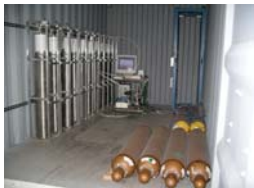
200 kg enriched xenon gas continuously monitored for leaks.
