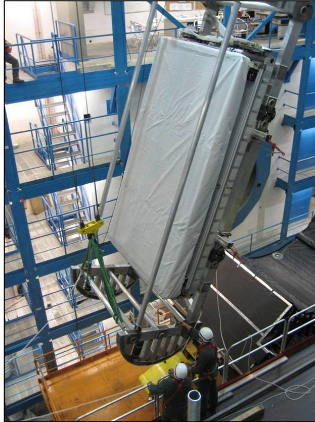
Thin Gap Ch 1 installation in UX15 – for EC trigger
