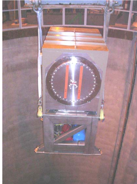
Being lowered and
