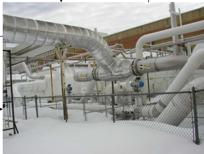
Cold Boxes (Heat Exchangers – Energy Exchange)
