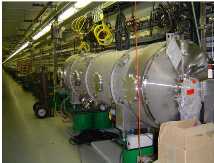
Cryomodule during Installation
