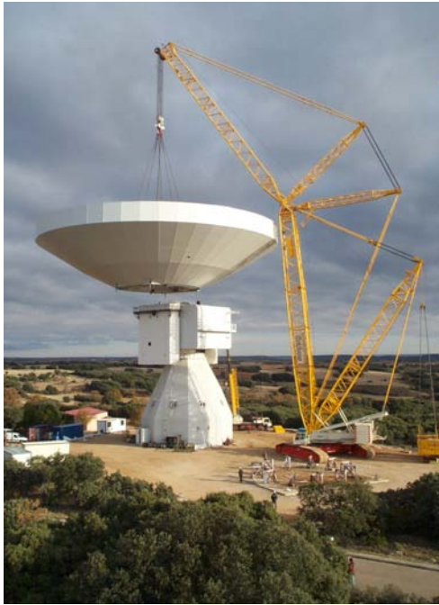
Figure 8: Lifting the main reflector of the 40 meter IGN radio telescope.
