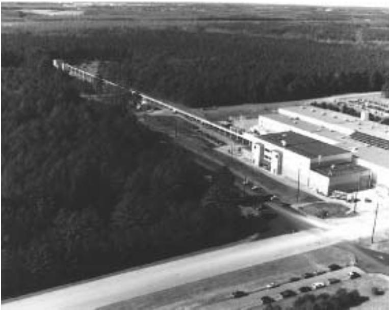
Figure 8: Aerial view of the X-Ray Calibration Facility at NASA's Marshall Space Flight Center. The large building to the right houses a thermal-vacuum chamber. A 525-m evacuated tube connects the chamber to various X-ray sources.
