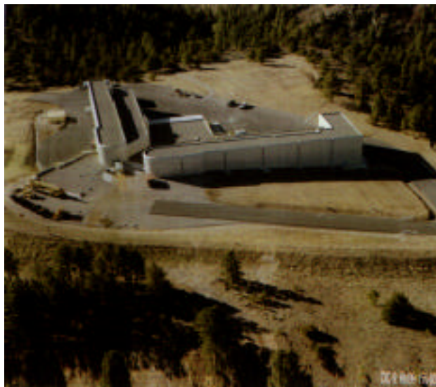
Fig. 10. The DARHT facility at LANL. The axes of the two radiographic machines are at right angles.
