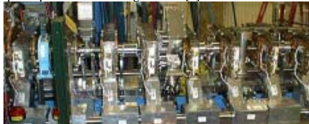
Figure 1. Shown above are the initial 8 quadrupole magnets, 2 steering magnets, and the initial beam diagnostic instruments in the quadrupole-magnet lattice.
