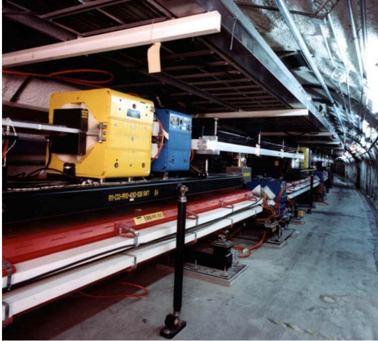
Figure 2-2: The PEP-II storage ring. The upper ring is the low energy positron ring and the lower ring is the high energy electron ring. Courtesy of Stanford Linear Accelerator Center.
