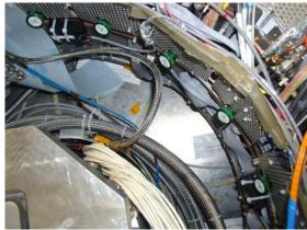
Figure A.4: Two sew sensor installed at 12 o'clock and 3 o'clock positions.
