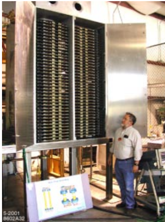
Figure 4.11: Full-scale modulator prototype with drivers installed.
