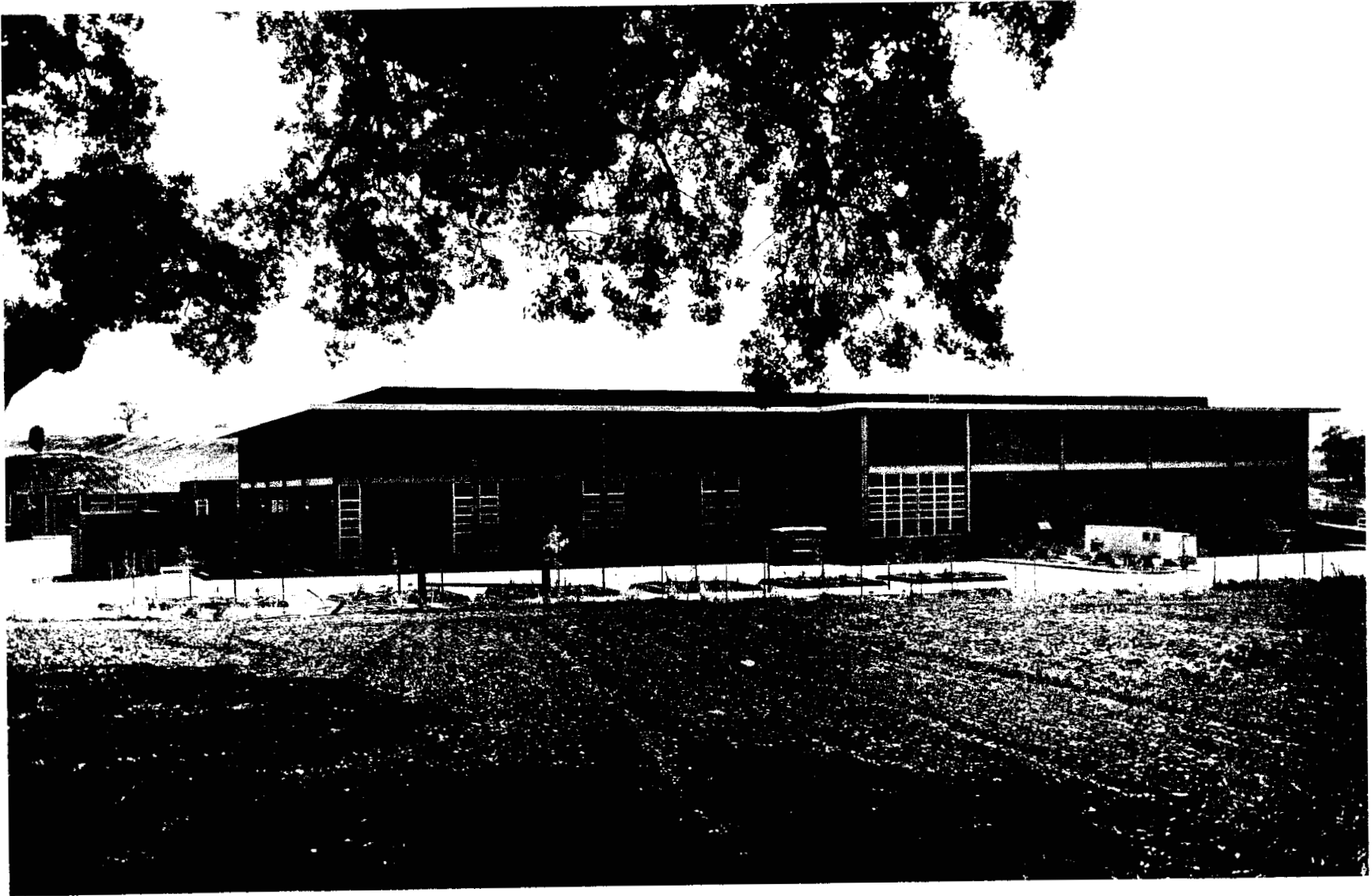
FIG. 4--General Services Building, front entrance.
