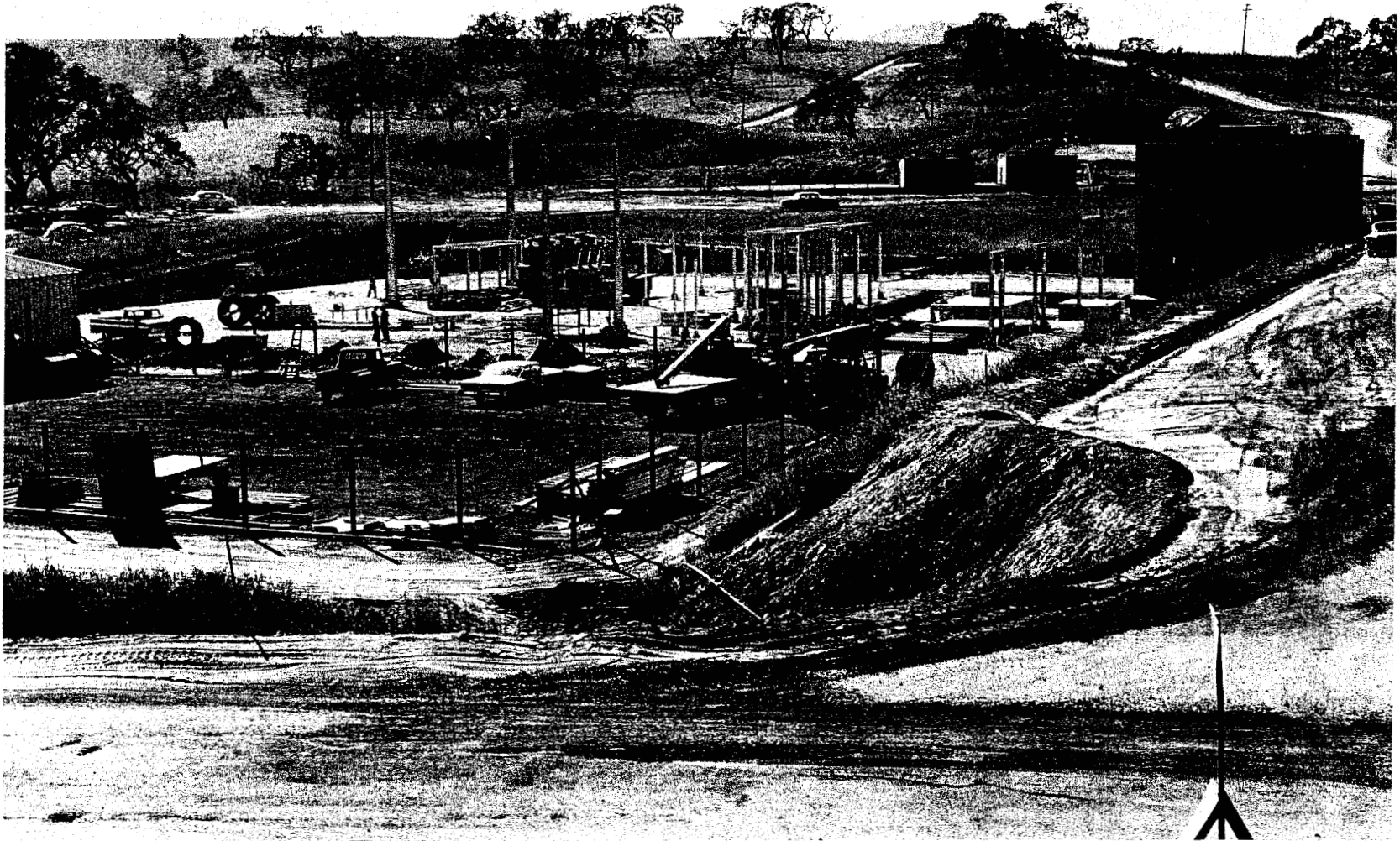
FIG. 6--220-kV master receiving substation and switch house.
