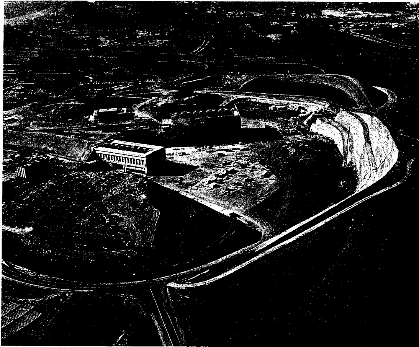
Fig. 1--Target area and end stations, looking northwest.
