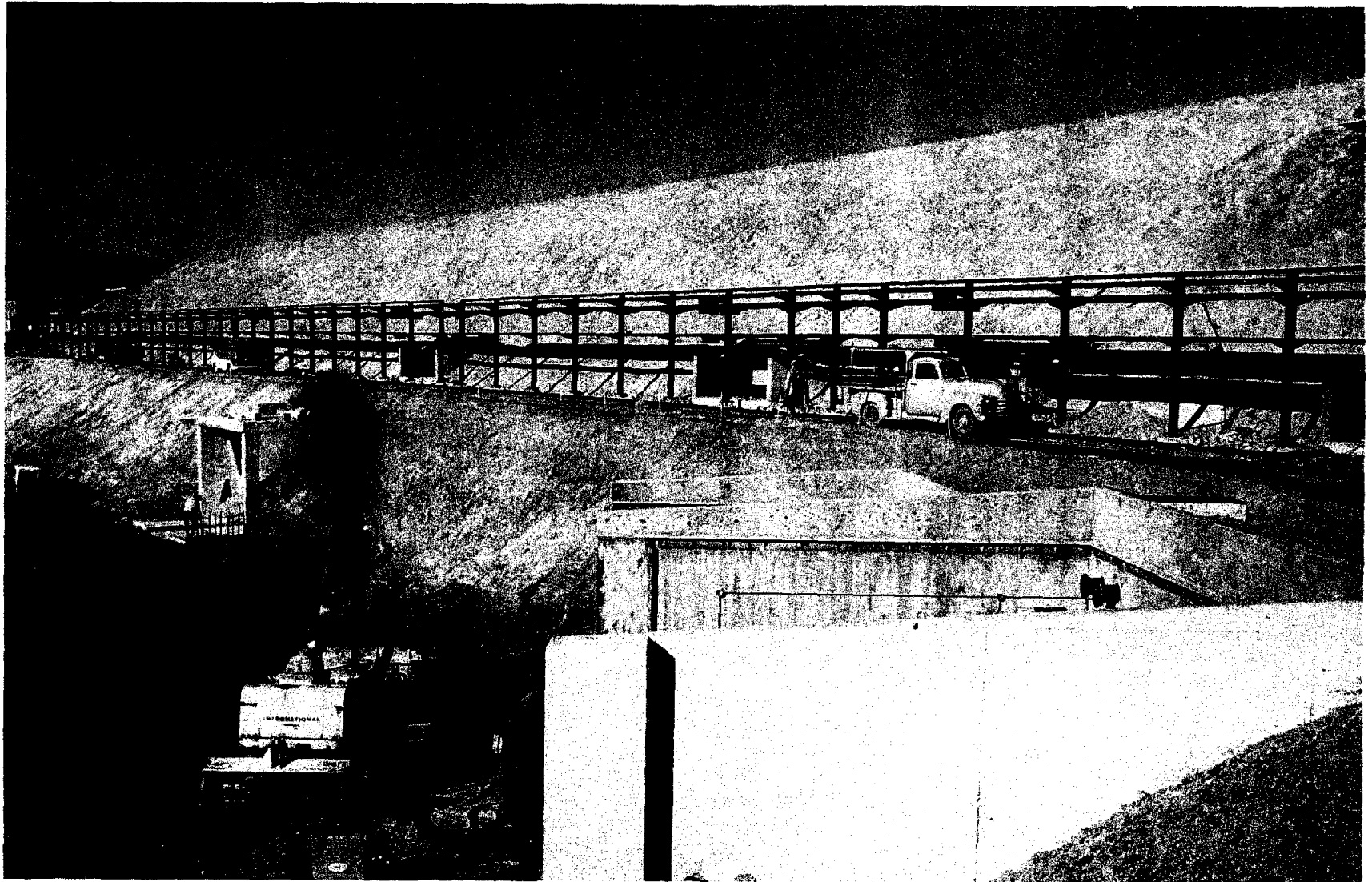
Fig. 4--Instrumentation and control support structure; south side of Beam Switchyard fill
