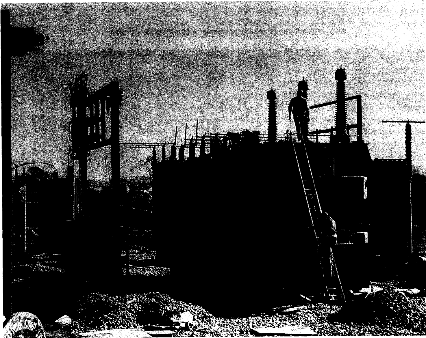
Fig. 2--220/12.47 kV transformer at master substation
