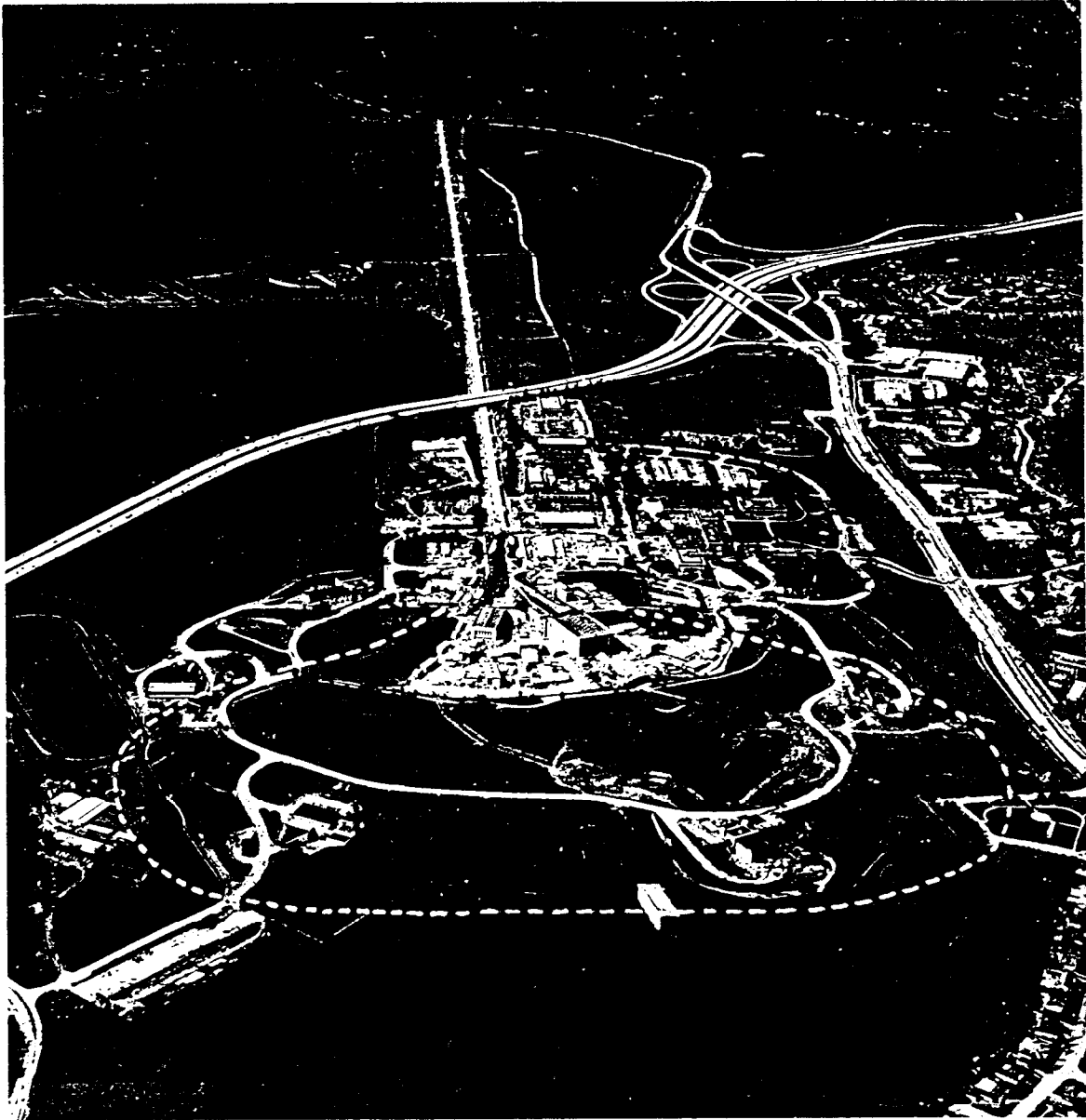
Fig. 8 SLAC Site - looking west. PEP IR Halls & SLC Collider Hall are in foreground. Artificial sight berm lies between above structures and Sand Hill Road, Sharon Heights & Stanford Hills.
