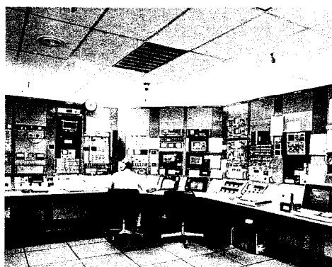
Fig. 2. The PEP main console area located in the PEP Control Room (PCR).
