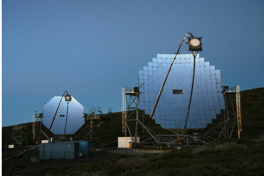
Figure 1: The MAGIC 17m imaging atmospheric Cherenkov telescopes at the Roque de los Muchachos Observatory, La Palma, Spain. Both telescopes are 85m apart. Image copyright: Robert Wagner.
