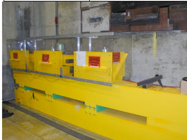
Figure 2: Photo of stabilization demonstration system.
