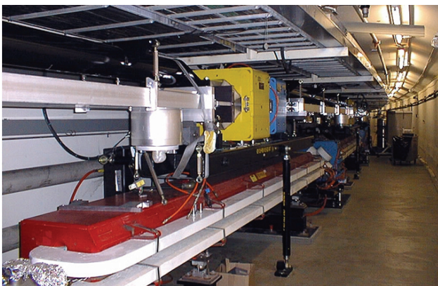
Figure 1. View of the PEP-II tunnel. The LER beam line is above the HER beam line.
