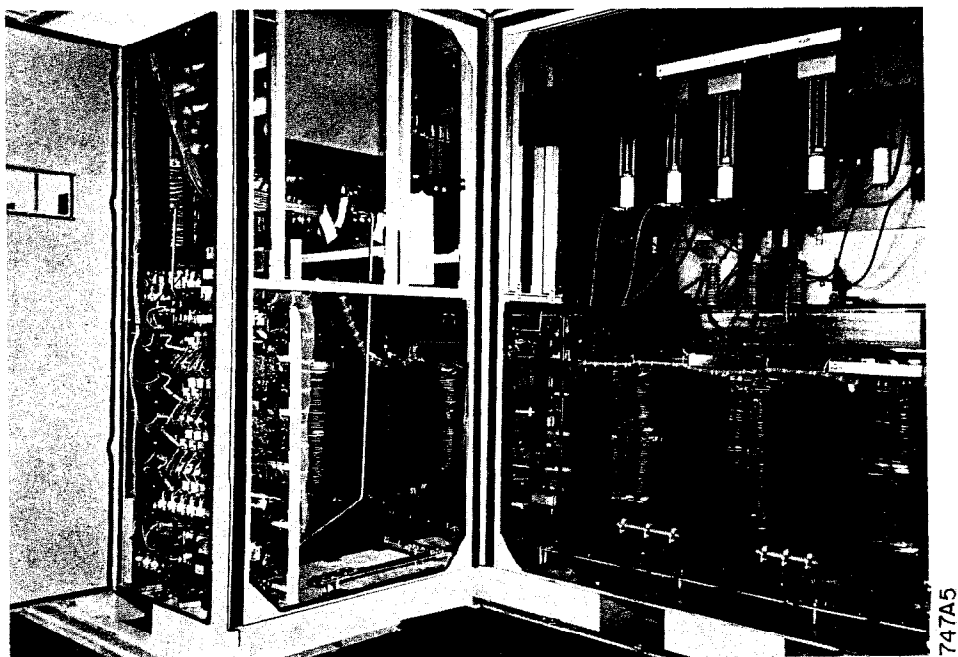
FIG. 4 -- 5800 kW POWER SUPPLY RECTIFIER CABINET 2 REMOVED.
