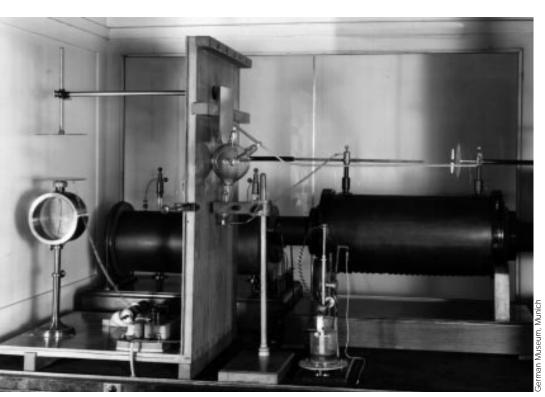
Roentgen's apparatus for studying the ionization of air by X rays, 1906.
