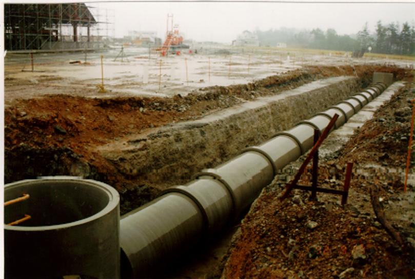
Fig.11. Drain pipe before tunnel floor construction.
