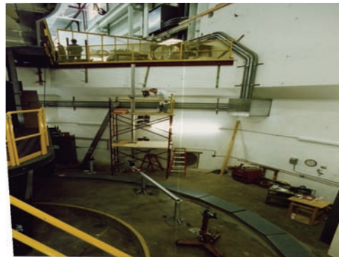
Figure 4. Installing the S800 spectrometer using a tooling dock.
