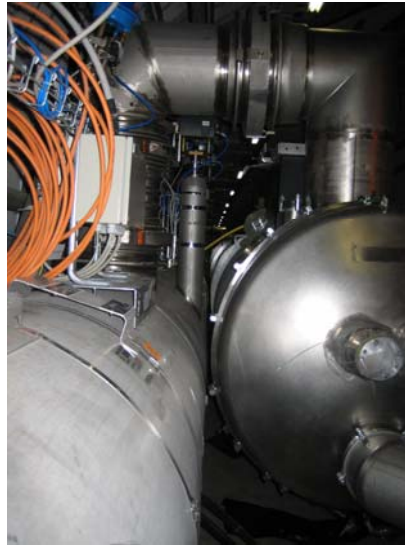
Figure 9: The QRL line with the jumper connection
