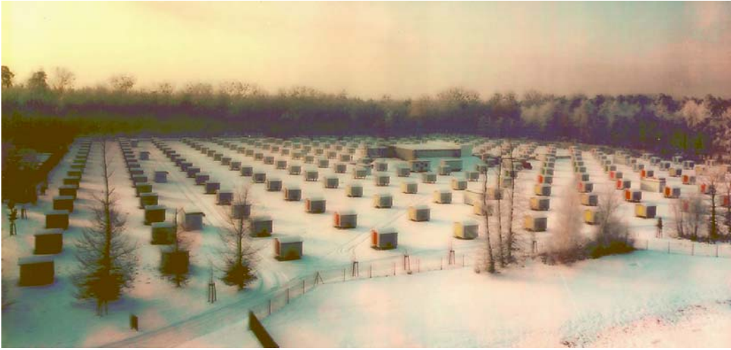
Figure 1: View of the KASCADE cosmic ray experiment [5]. The small huts house detectors for electrons and muons. The calorimeter is the larger building in the background.
