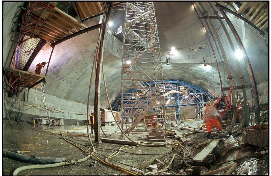
Underground construction at the ATLAS cavern
