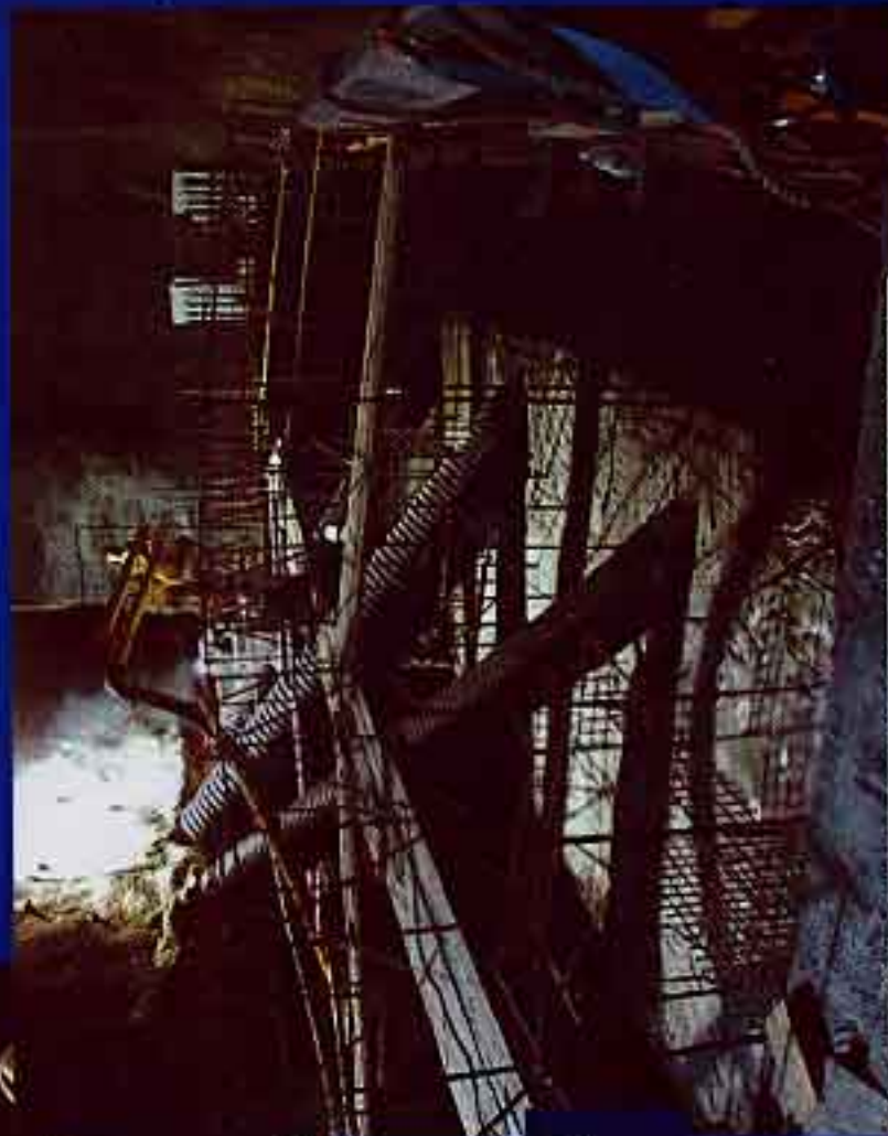
Point 5 - Installation of fibre optic ducts in the pillar (level -2.3m) - June 15, 2001
