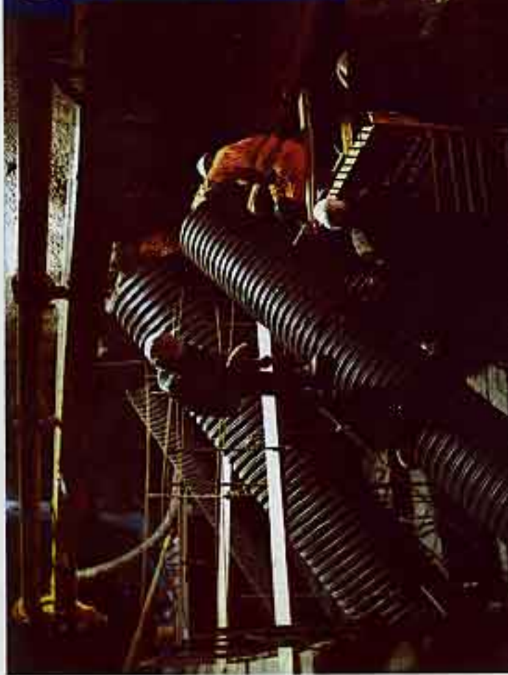
Point 5 - Installation of fibre optic ducts in the pillar (level -2.3m) - June 15, 2001
